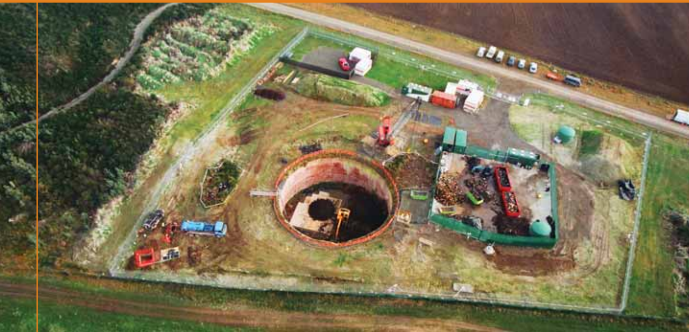
Aerial of the remediation site.
