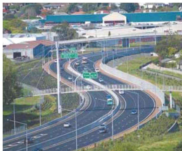
Award Winning Extension Section of the SH20 Mt Roskill Project.
