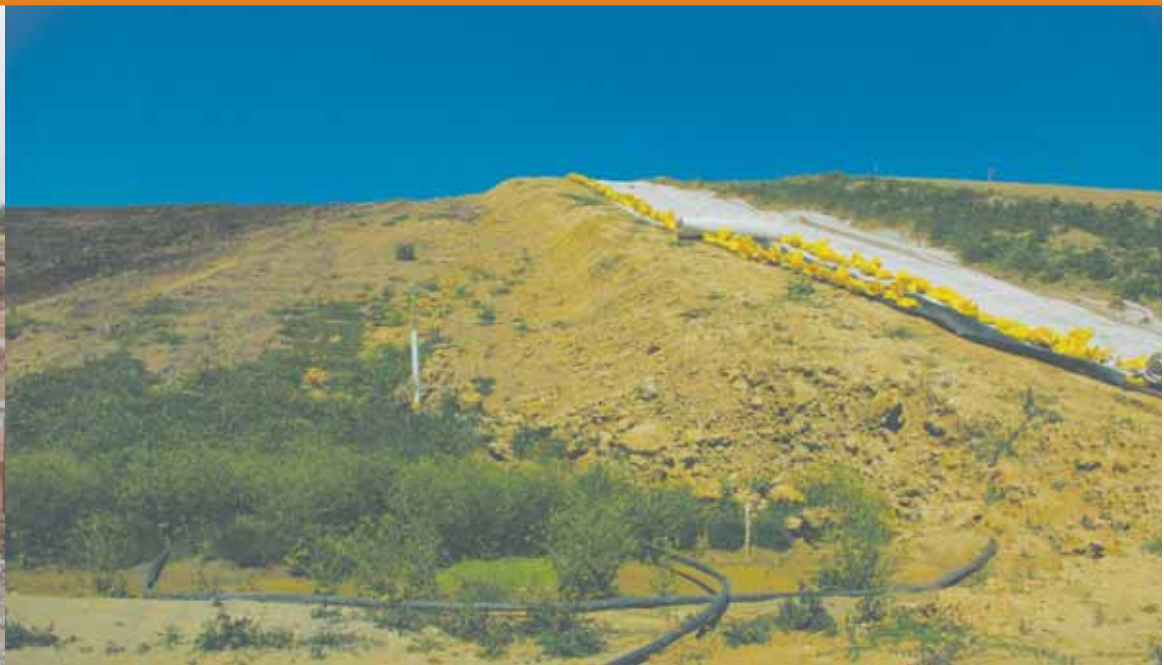
CALM showing capping layers.
