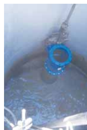
The Macmasters Beach refurbished pump station (left) with new wet well pumps, pipe work, fittings, protective coating and instrumentation (right).
