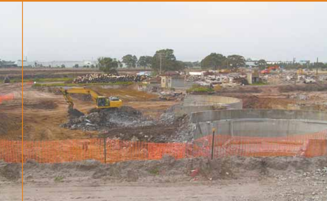
Trade Waste Treatment Plant during demolition.
