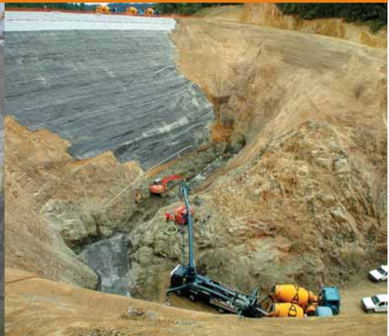
Cosseys Dam, New Zealand.
