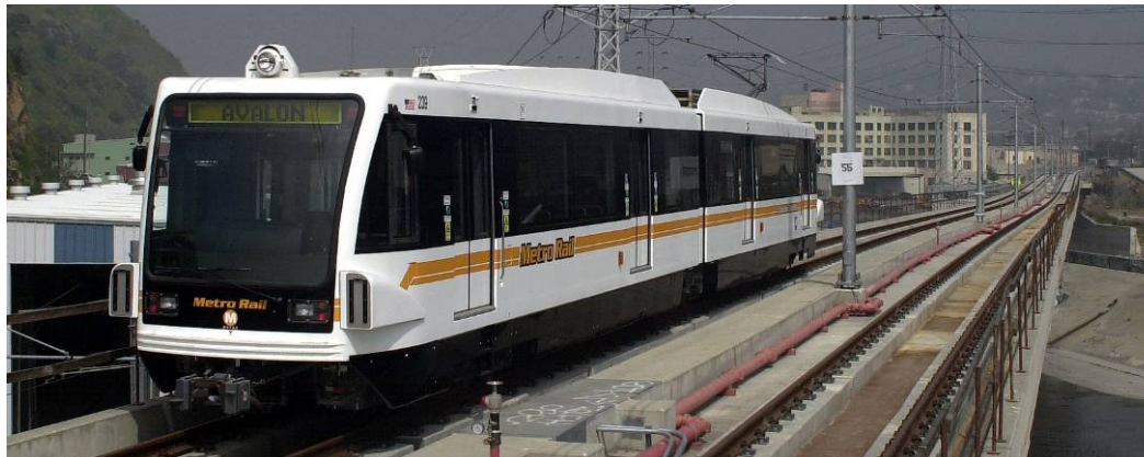
Los Angeles Metro Gold Line
