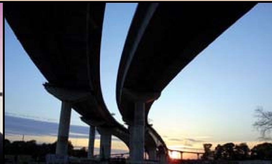
New James River Crossing- Virginia High-rise bridge, clear waterway structure
